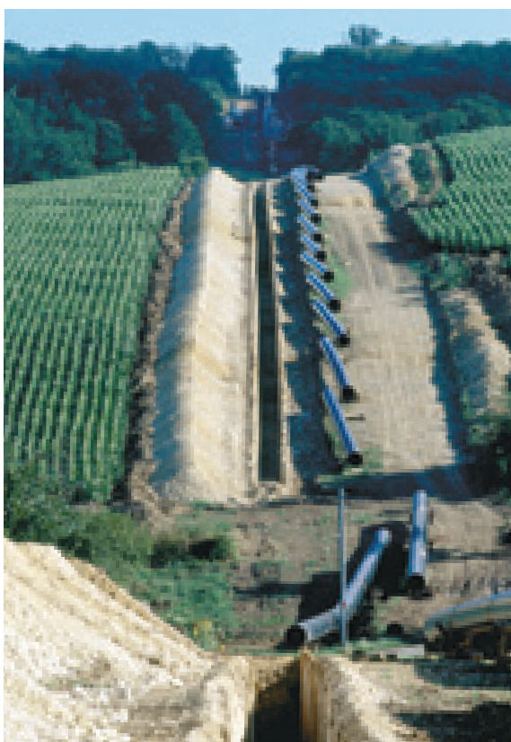
Stringing tubes for the loop in southwestern France.
