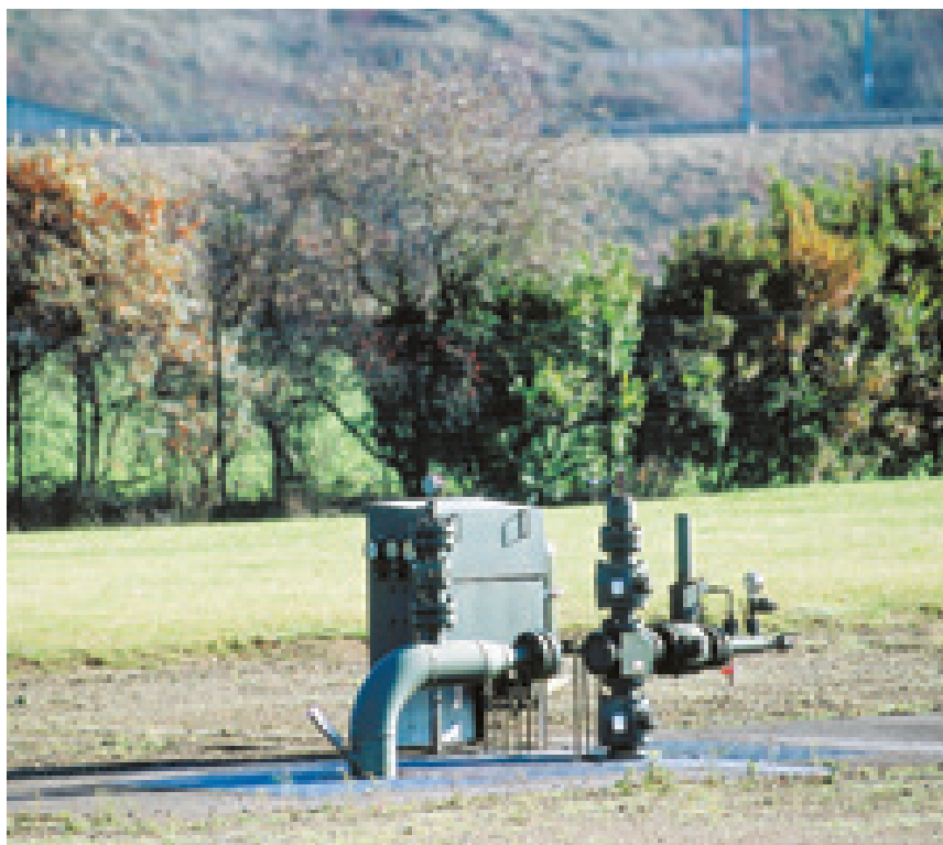
Wellhead of an underground storage facility.
