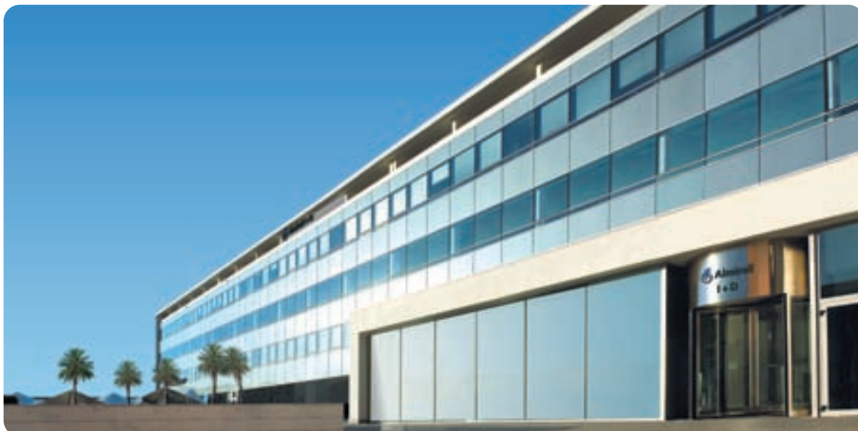
Almirall's R&D Centre in Sant Feliu de Llobregat (Barcelona, Spain)
