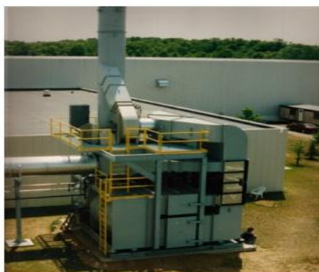
25,000 SCFM Catalytic Oxidizer with preheat exchanger (8 Weeks Deliv.)
