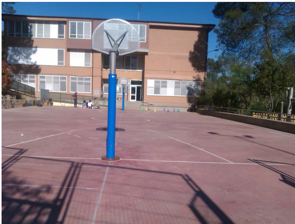
Millora 16: pista exterior irregular
