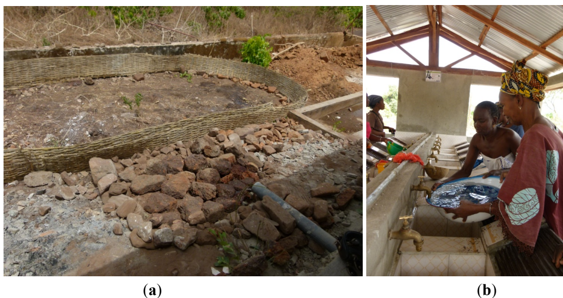
Figure 9. (a) Filter system and Moringa oleifera intensive bed; (b) Local women using the new washing facilities.
