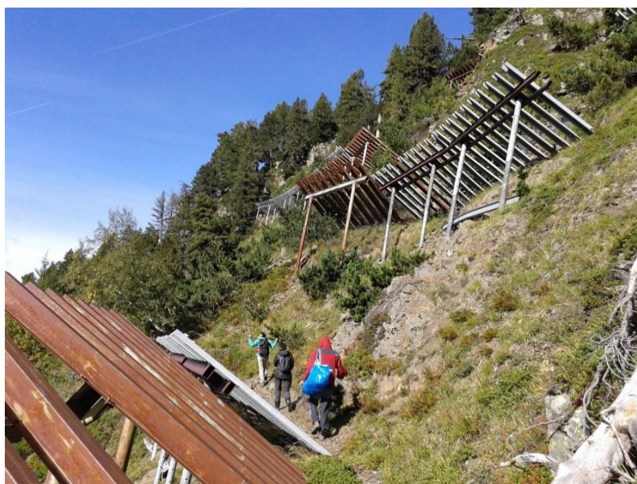
Figure 1. Anti-avalanche structures in Thiel corridor above Barèges.
