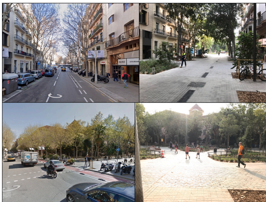
Fig. 2. Consell de Cent Street before and after pedestrianisation (source: Google Street View/authors).
