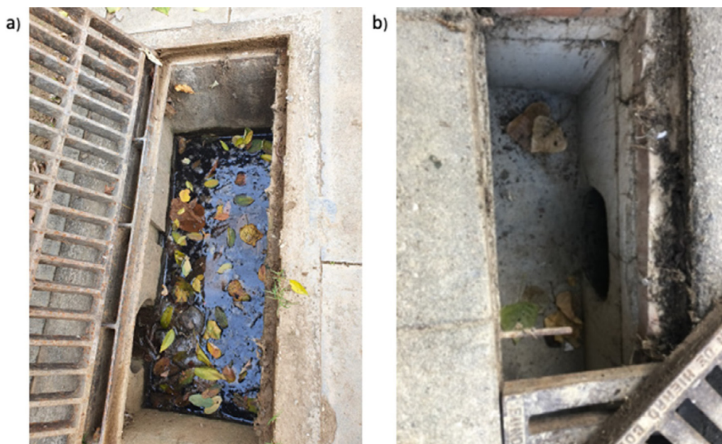
Fig. 3. Panel a) depicts an unmodified storm drain with stagnant water, and panel b) depicts a modified storm drain. Source: We obtained photos from [17] with permission for re-use.
