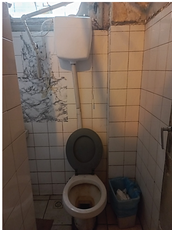
Figure 13. Disposal bin in public toilet in Rio de Janeiro.
