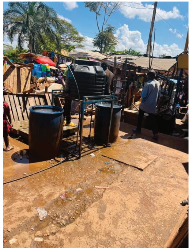
Figure 5. Hand washing station in a public toilet outside a market in Kampala.
