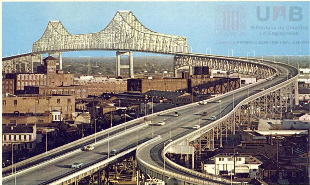
New Mississippi River Bridge
