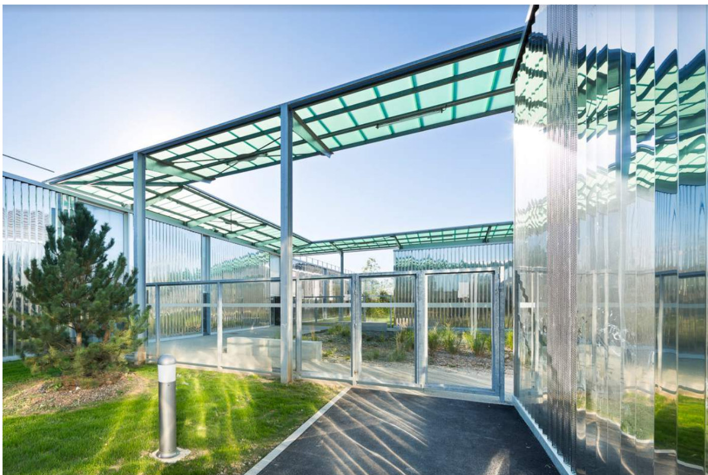
CFA de Brétigny , Brétigny-sur-Orge, France; ©ARCHI5 Aperam Stainless Steel used: Aperam 304 with Uginox Bright finish
