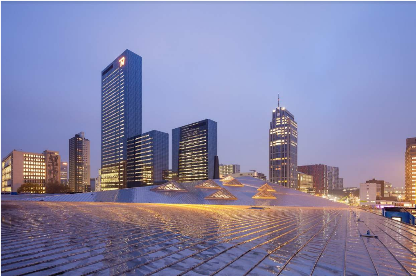
Rotterdam Central , Netherlands; © Jannes Linders; Stainless steel used: Aperam 16L Uginox Mat
