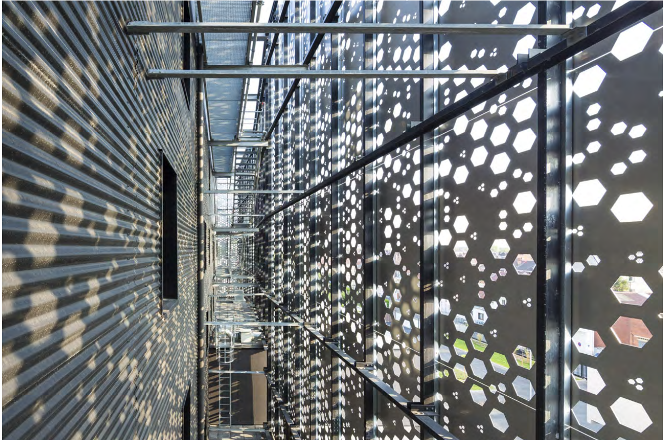
Conservation centre for the departmental archives of the Nord, Lille, France; de Alzua+ / ZigZag Architecture © Sergio Grazia Aperam stainless steel used : 304 with Uginox Mat surface finish
