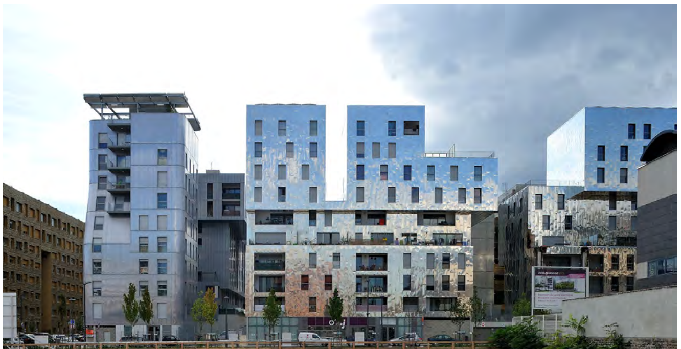
Apartment building "Lyon Islands ", Lyon - France; © Massimiliano & Doriana Fuksas Aperam stainless steel used : Uginox Bright Nuance: 304/1.4301
