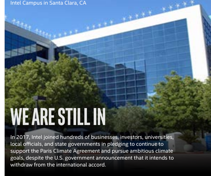
Wind Power Installation Intel Campus in Santa Clara, CA
