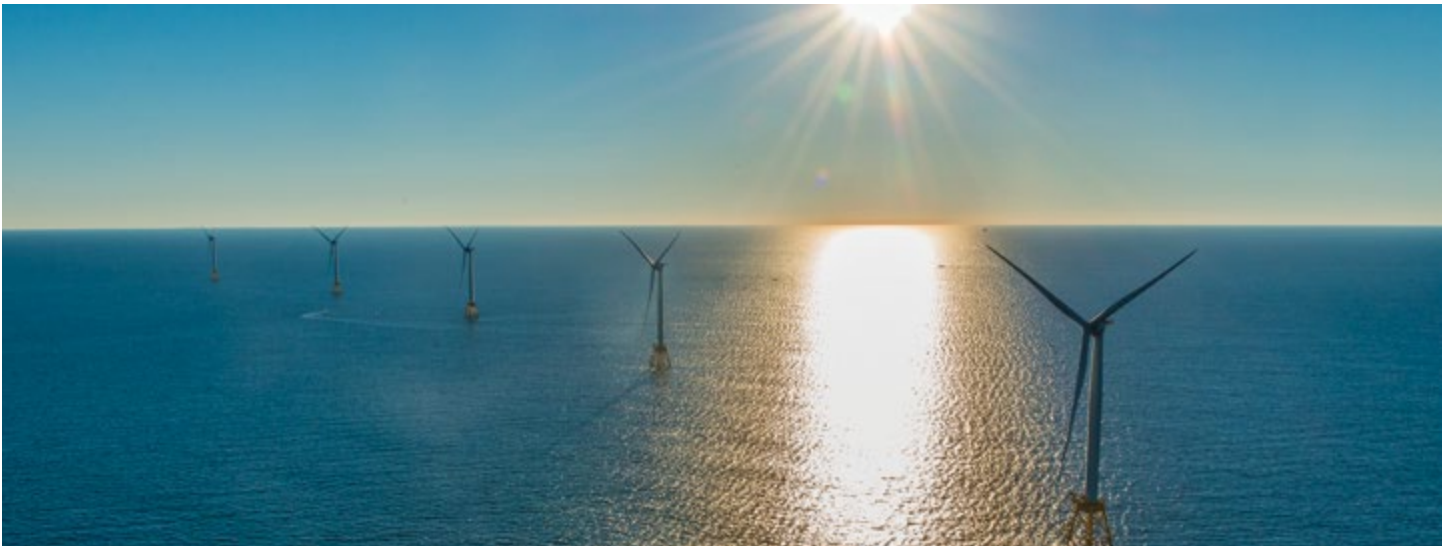
Block Island Wind Farm
