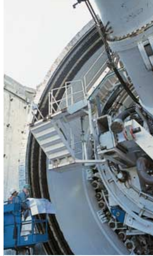
Tunnel-boring operations with a TBM have started on the A86 motorway around the west of Paris. The first toll-paying section will be opened to the public in November 2004.
