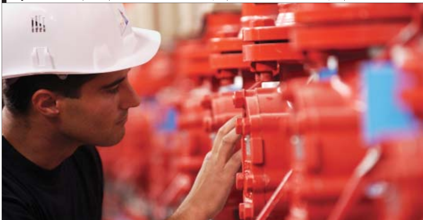
Design and installation of fire protection systems for the Deret warehouse in Orléans: 18,000 sprinkler heads were installed in an area of 55,278 square metres
