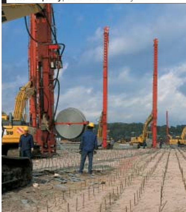
Vacuum compacting prevents the soil from settling
