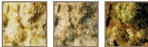
Right: the Digue Verte® (Grand Prize). Above: the roughness of the facing on the submerged part of the Digue Verte® fosters rapid colonisation by marine flora and fauna.
