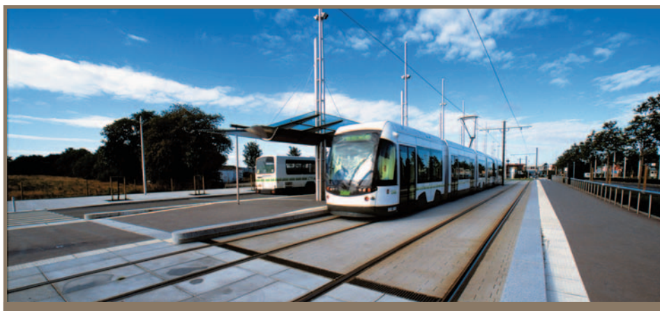
Eurovia, which has worked on many tram projects in France (such as Nantes, above) and abroad, won the contract to build the third tram line in greater Grenoble.
