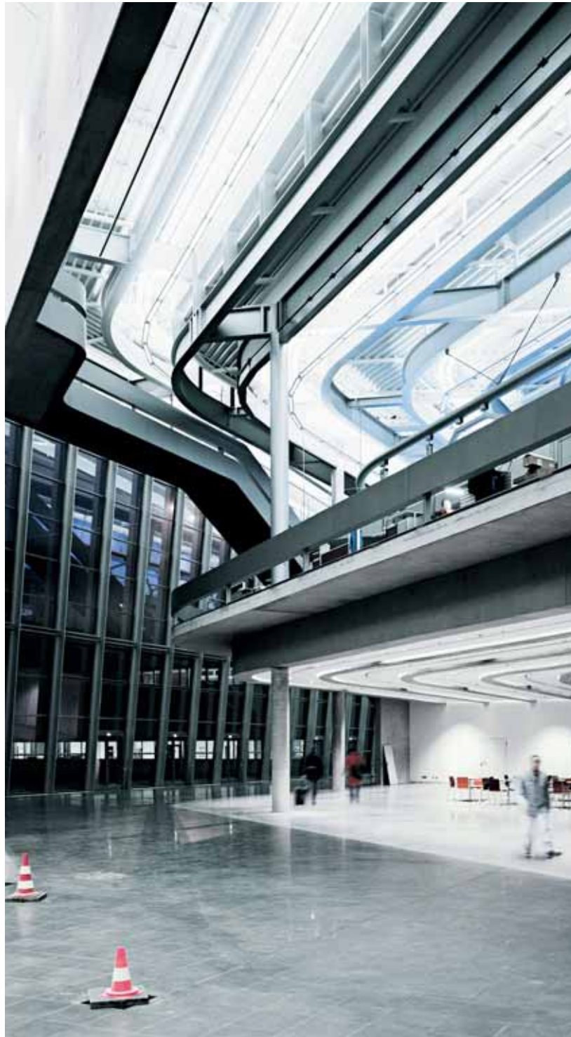
A vision becomes reality: very soon after construction work started, the Venice Biennale 2002 included the BMW Group and its exciting design of the central building for the Leipzig plant.
