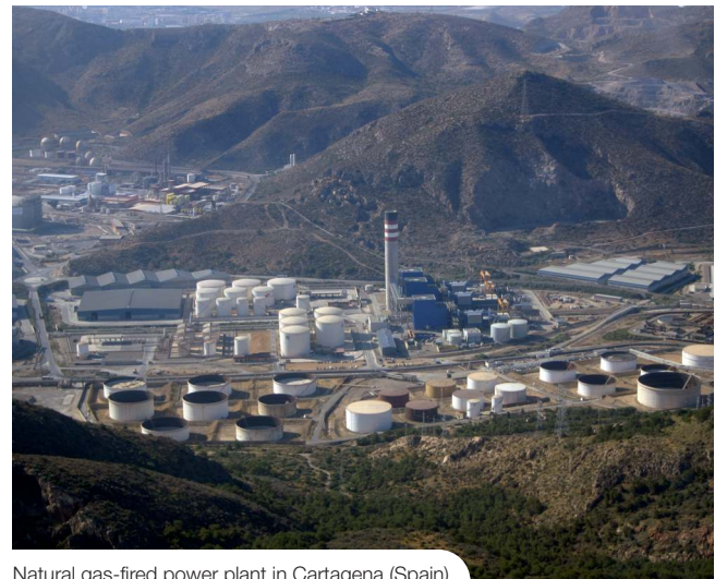
Natural gas-fired power plant in Cartagena (Spain)
