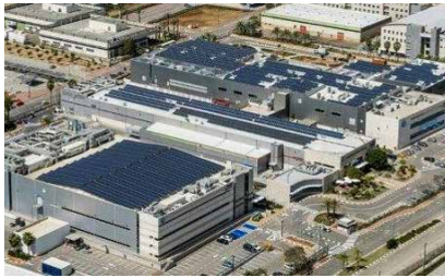
Solar panel installation at HP Kiryat Gat, Israel
