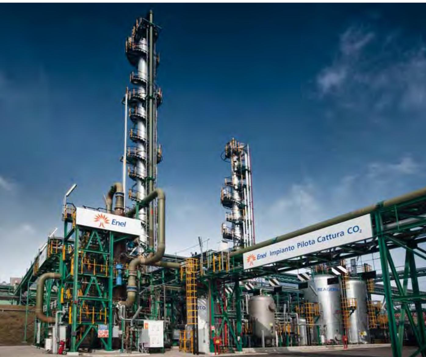
demonstrating carbon capture and sequestration (CCS) technologies, focusing on capturing coal plants' CO<sub>2</sub> emissions (post-combustion capture), on innovative oxygenated coal combustion technologies, and technologies for the gasification of fossil fuels (pre-combustion capture) and on CO<sub>2</sub> storage solutions.
