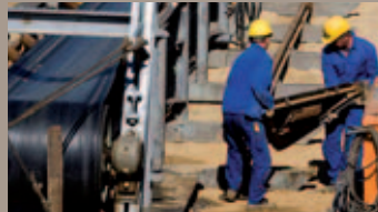
Workers on a construction site
