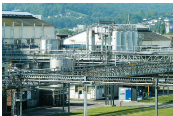
Elbeuf industrial site (France).
