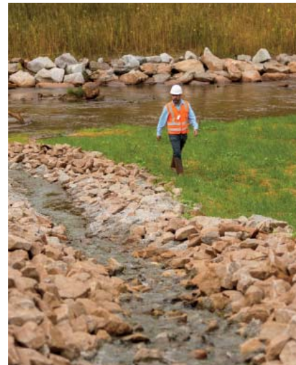
Reinforcement of tributaries and stabilisation of river margins.
