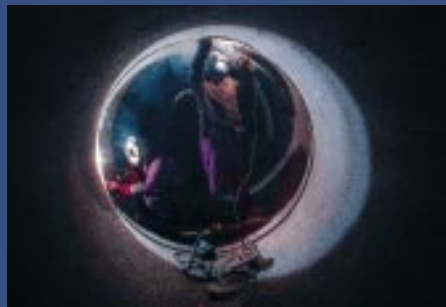
Main picture: Giant tunnelling machine used to drill the mile long underground stormwater tunnel at Hastings arrives in sections at Hastings beach. Far left: Barge carrying the drill from Germany arrives at Hastings. Left: Welding the outfall pipe for the new Dover and Folkestone waste water treatment plant.
