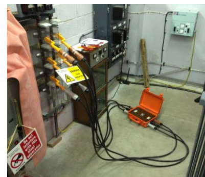
Figure 7 LV Jumper Applied
