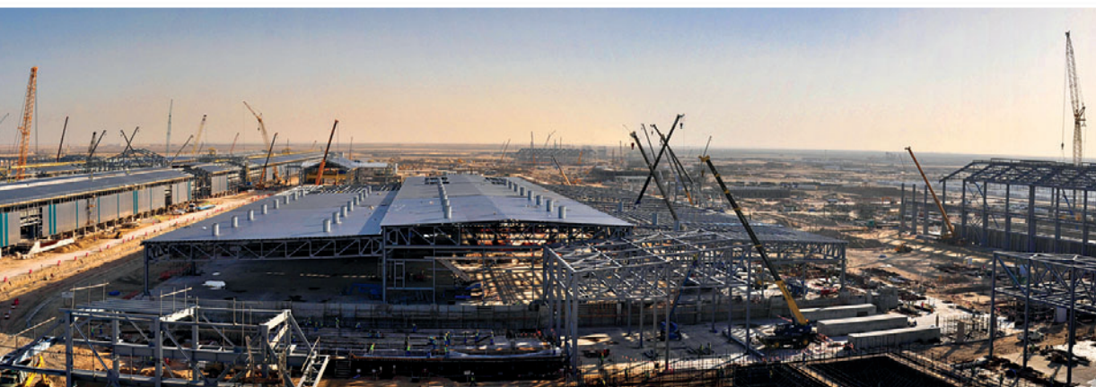
Construction progress at the Ma'aden-Alcoa integrated aluminum complex, October 2011
