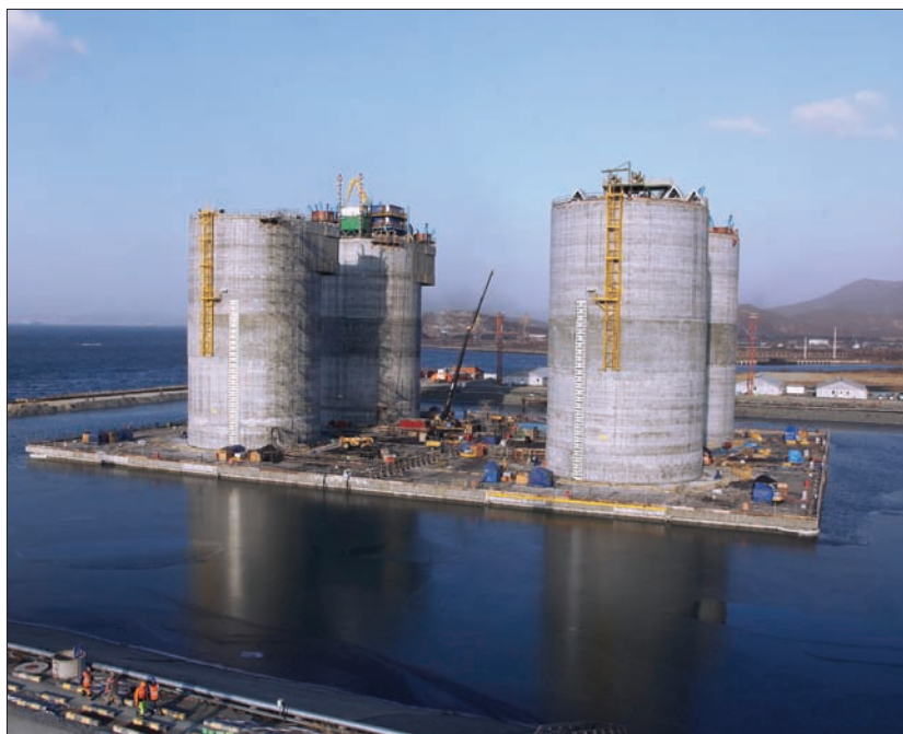
We achieved mechanical completion of the Arkutun-Dagi offshore platform concrete gravity-based substructure (GBS) in December in far east Russia.
