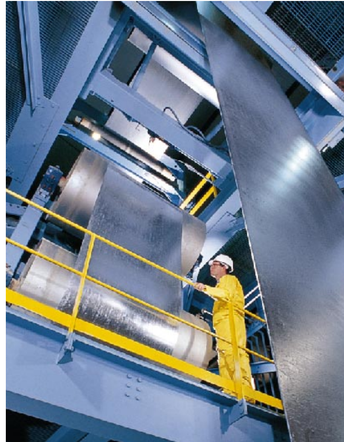
GE's Bill Erichson inspects a roll of galvanized steel coil at the Nucor mill in Hickman, Arkansas, where GE Industrial Systems provided a complete solution: drives, motors, switchgear, control centers, software, and related equipment and services.
