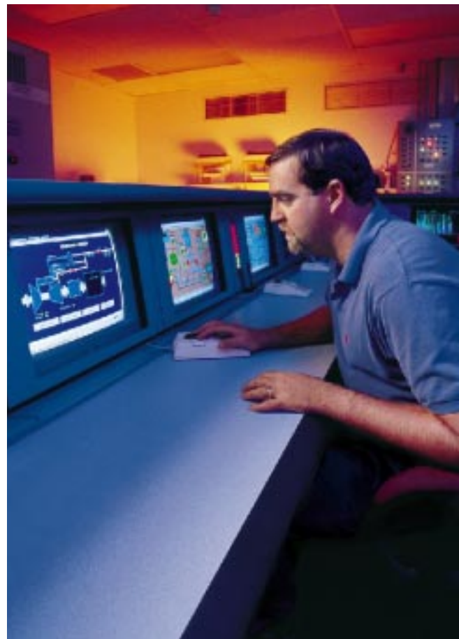
Jim Soutter checks the performance of a GE gas turbine at the Cardinal Cogen Power Plant. GE Energy Services has a multiyear service contract at this plant, which provides electric power, heat, refrigeration and air conditioning to Stanford University.
