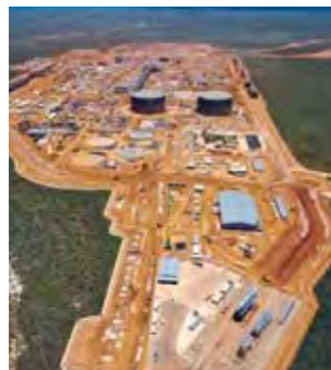
Gorgon Project facilities on Barrow Island.
