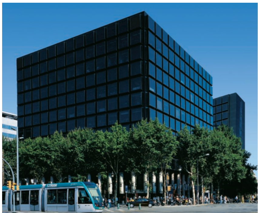
AVINGUDA DIAGONAL, 609-615, BARCELONA
