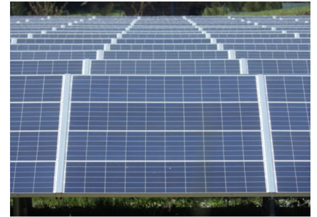
Solar array installation at IBM’s data center in Vaux-sur-Sûre, Belgium.
