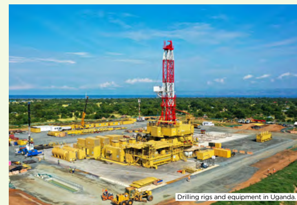
Drilling rigs and equipment in Uganda.
