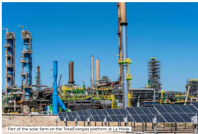
Part of the solar farm on the TotalEnergies platform at La Mède.
