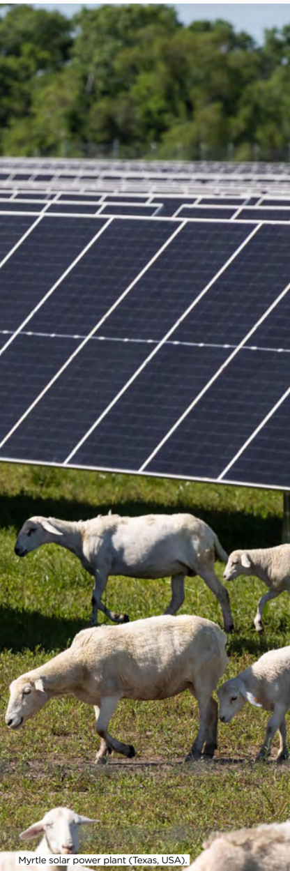
Myrtle solar power plant (Texas, USA).
