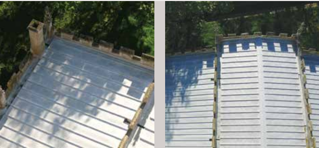
The stainless church roof has excellent resistance to high wind, is lead-free and inert.
