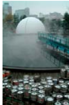
Wastewater treatment plant at Leuven showing the bio-gas holder.
