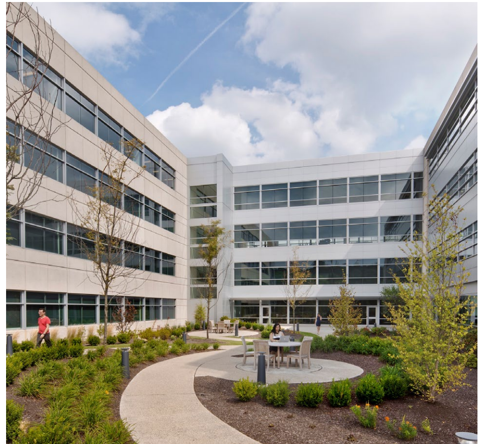
Honeywell, Morris Plains, New Jersey
