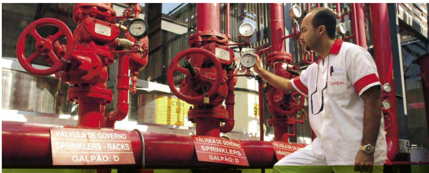
► Inspection of our fire sprinkler system in our Rio de Janeiro (Brazil) factory.
