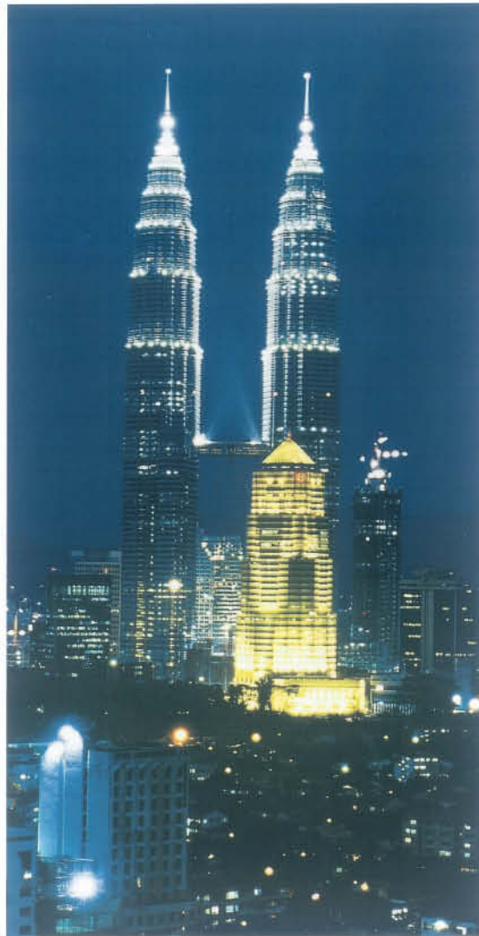
The Petronas-Towers in the Malaysian capital Kuala Lumpur are lit by 180,000 Osram lamps. An electronic control system ensures energy-saving power consumption.
