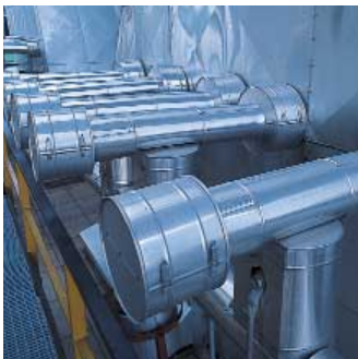
Flue gas sampling points on denitrification system inlet
