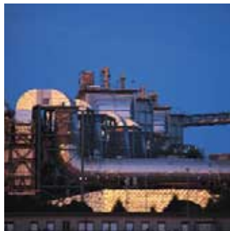
Desulfurizer inlet/outlet flue gas ducts
