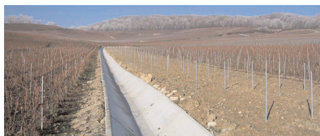
Example of hydraulic installation.
