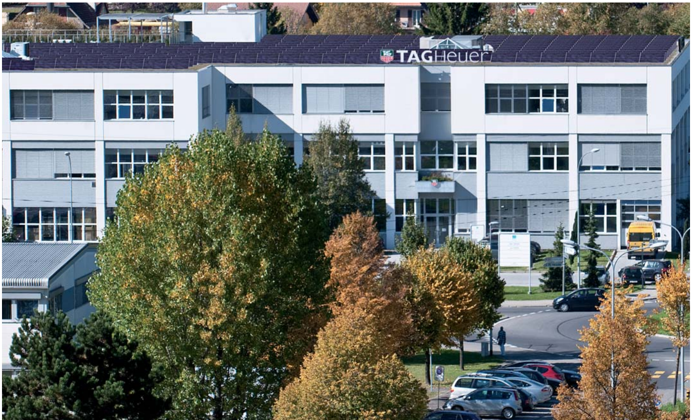
TAG Heuer is installing 750 m 2 of photovoltaic panels on the roofs of its buildings in La Chaux-de-Fonds.
