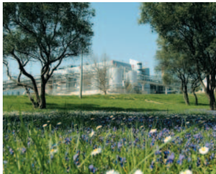
Aramon chemical manufacturing facility.
