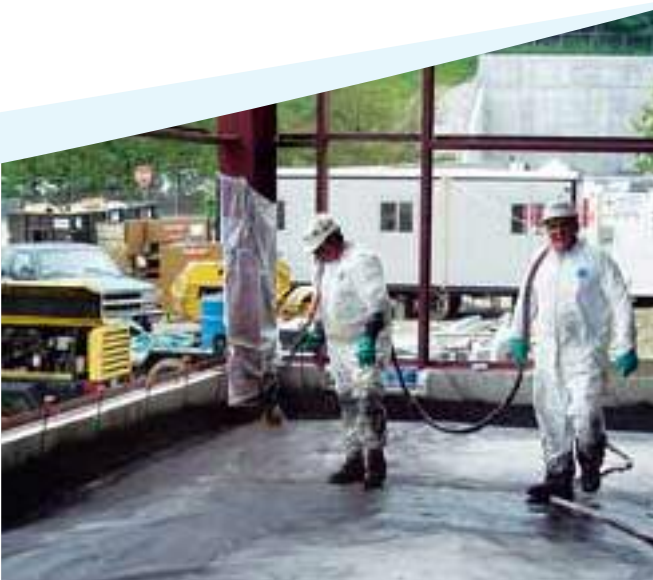
Application of impermeable vapor barrier to mitigate potential exposure pathways
