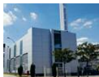
New boiler room and gas effluent treatment unit at the Vitry Production Center
