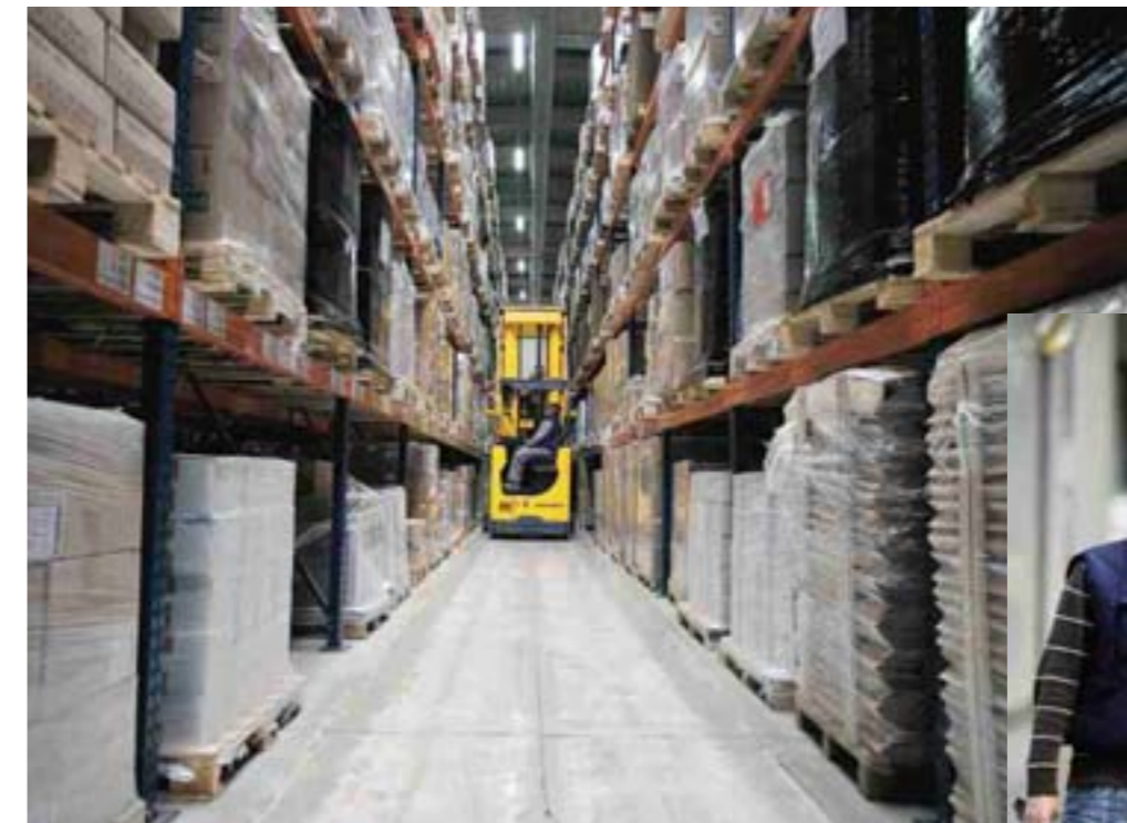
Distribution site at Croissy-Beaubourg (France).
