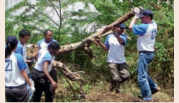
Speedy, unbureaucratic assistance: cleaning-up work following the devastating floods
