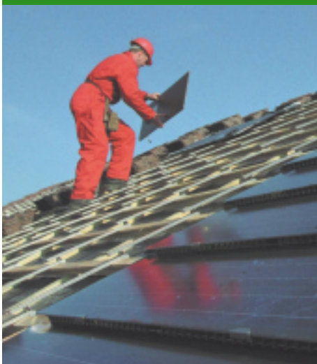
ROOFING | Installing photovoltaic systems
