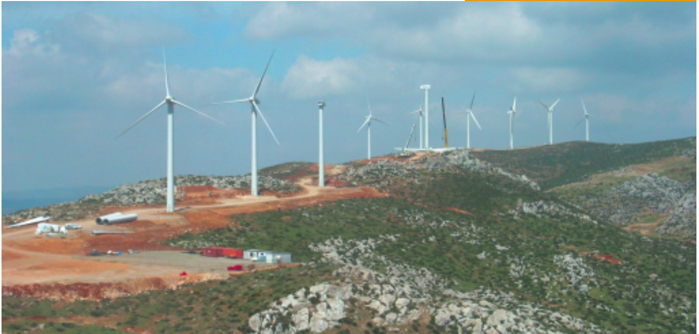
MOROCCO | Wind farm under construction at the Tetouan II cement plant
