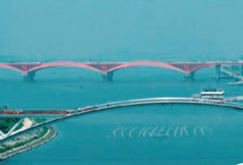
In the foreground, footbridge of Seonyu in Korea, realized with Ductal
