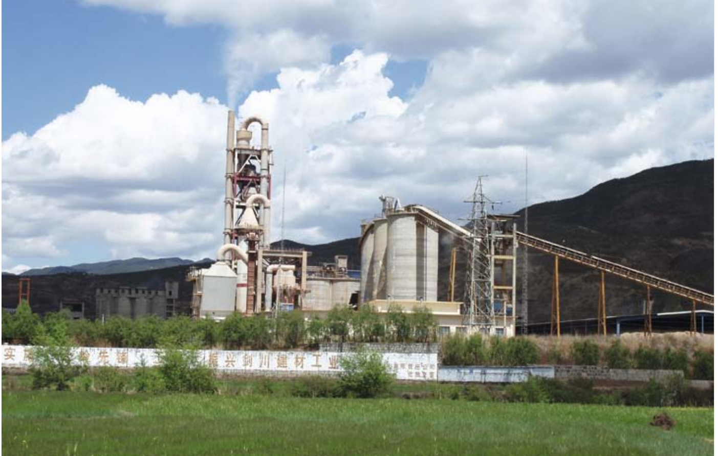
Jianchuan cement plant, China. © Lafarge Medialibrary - Xinping Zhang
