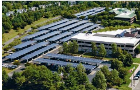
The award-winning photovoltaic system provides Munich Re in Princeton, USA, with green electricity from 12,000 square metres of solar panels.
