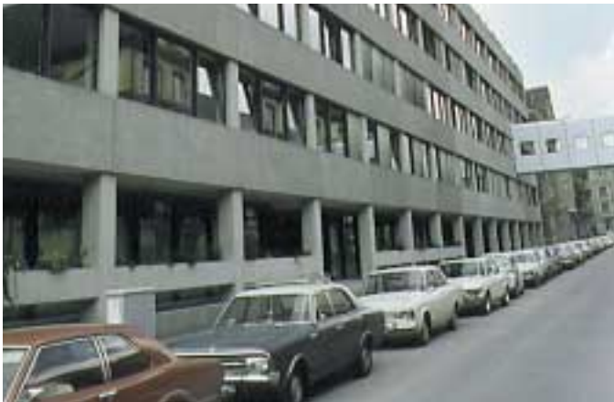
South 1 was completed in 1973 immediately after the oil crisis
